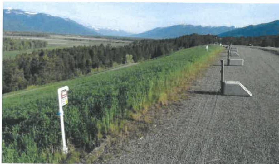
Photo 23. Completed Landfill Closure Cap and Seeding at Creston Landfill, B.C.
