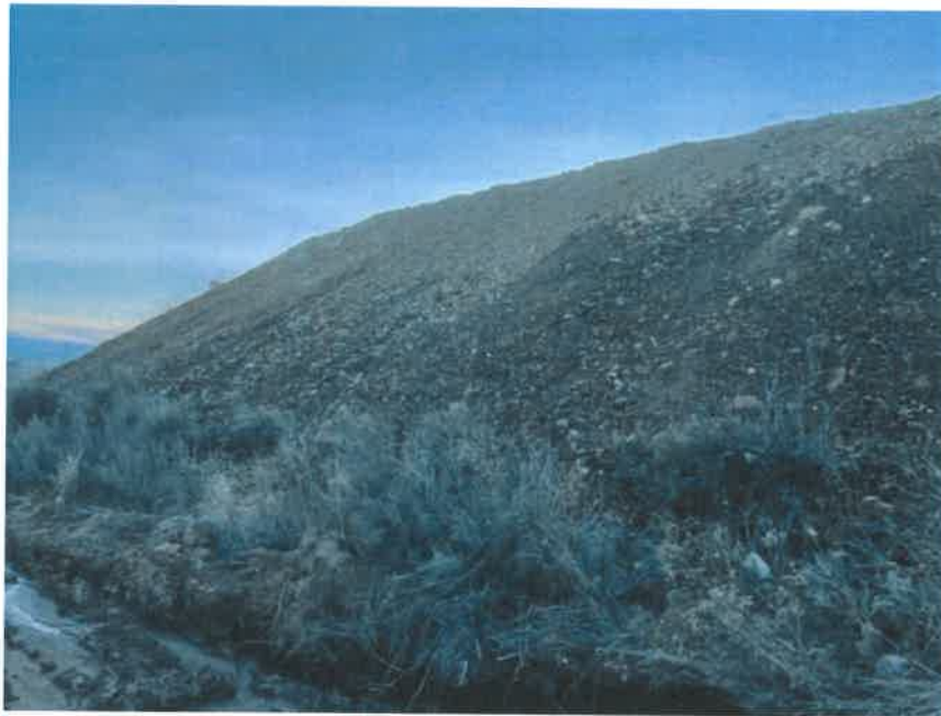
Photo 3. Steep Slopes covered with coarse gravel intermediate cover below lower bench road
