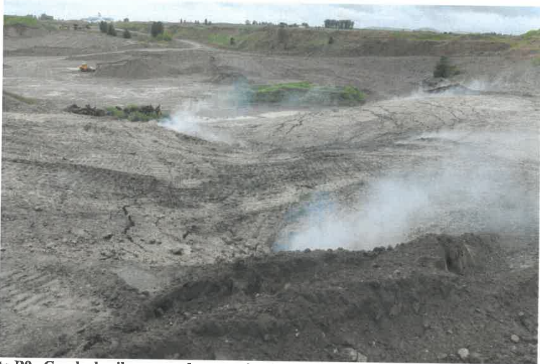
Photo B9. Cracked soil cover and vents releasing smoke at Lake County landfill Fire (2014)
