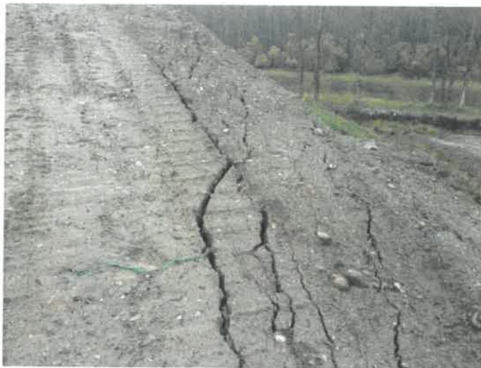
Photo 14. Soil Cracks developing in Berm at Skway Landfill
