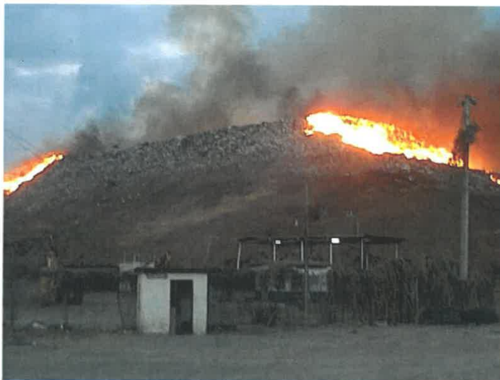
Photo B1. Cerro Patacon Landfill Fire (extinguished with Oxygen Suppression & Quenching Hot Spots)
