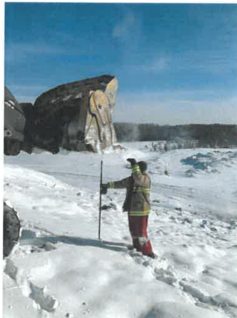
Photo 8. Bar Hole Punch Being Pushed with Track Loader
