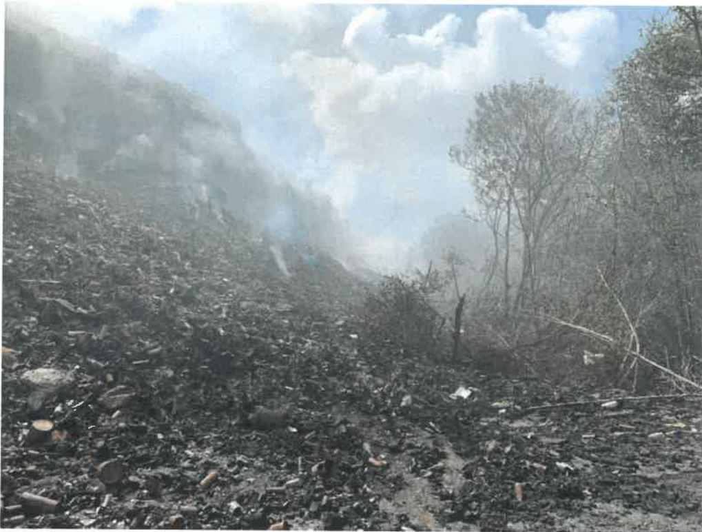
Photo B5. West Face of Roatan Landfill on Fire before regrading and soil cover
