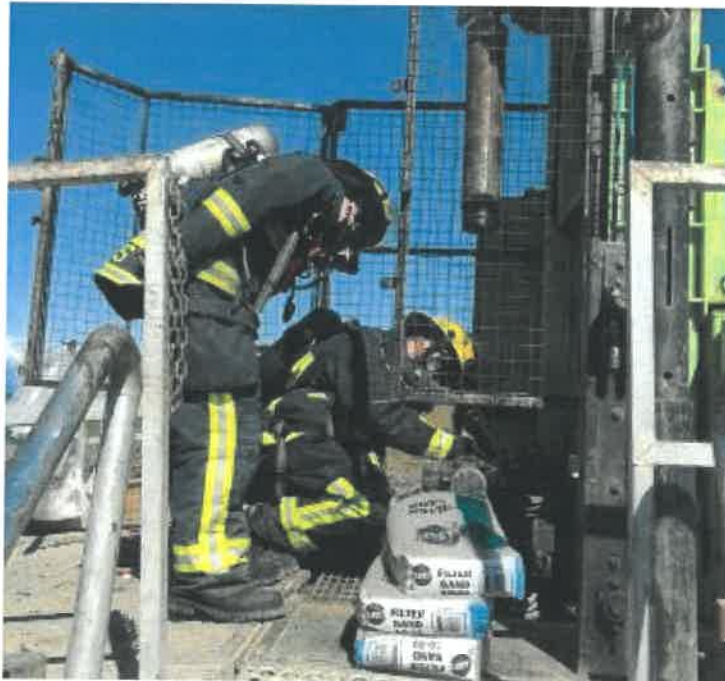
Photo 18. Delta Fire Assessing H 2 S Levels in Borehole with SCBA
