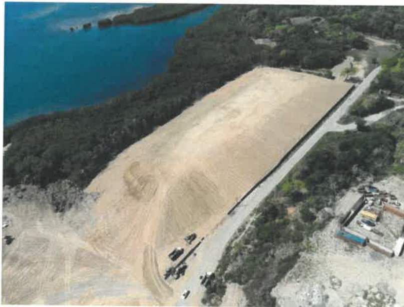
Photo B6. Roatan Landfill Regraded and capped per LFCI extinguishment plan.
