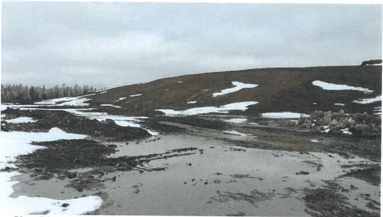
Photo B8. Edson Landfill with voids filled in and capped with 600 mm (2') of Clay (2019)
