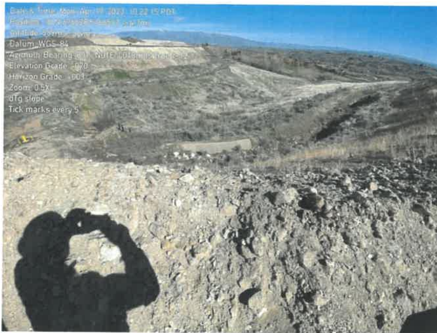
Photo 1. Site Photo from Lower Berm Looking to Northwest
